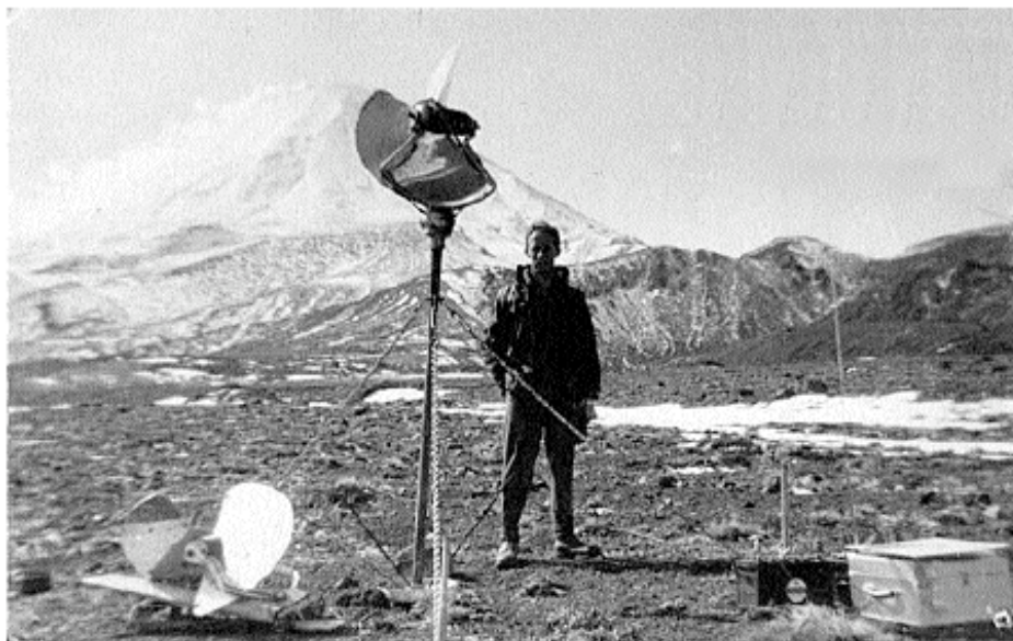
Fig 5a: Replacing wind powered generator damaged by storm in the explosion crater area located between Ngauruhoe and Ruapehu New Zealand. One explosion crater can be seen behind to my left in picture. Active Ngauruhoe Volcano in background to my left.
